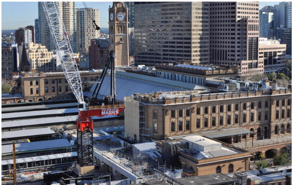
Marr's M1680D HLL is installed at Central Station to complete heavy lift and general construction requirements on above and below ground works associated with the redevelopment of Australia's busiest railway station.
