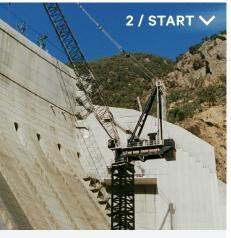
Backtrack to 1999, when Transfield was constructing a hydroelectric power station near Canberra in NSW, Australia and needed a solution for lifting heavy project components over a damn wall. We built the M1280D to do the heavy lifting in one lift, negating the need for the existing 'pass the parcel' series of cranes that were in place. It became the world's biggest tower crane.
