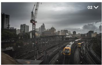
The heavy lifting capacity and reach of Marr's M2480D Heavy Lift Luffer (HLL) allowed construction partners, Laing O'Rourke, to install the crane at sufficient distance for the M2480D to remain in place during scheduled rail possessions for the installation of the bridge sections and during time-restrictive off-peak rail possessions at Australia's busiest railway station.
