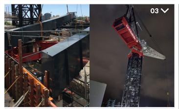
Marr's solution enabled the bridge sections weighing 60 tonnes to be assembled off-track and installed in a single lift.
